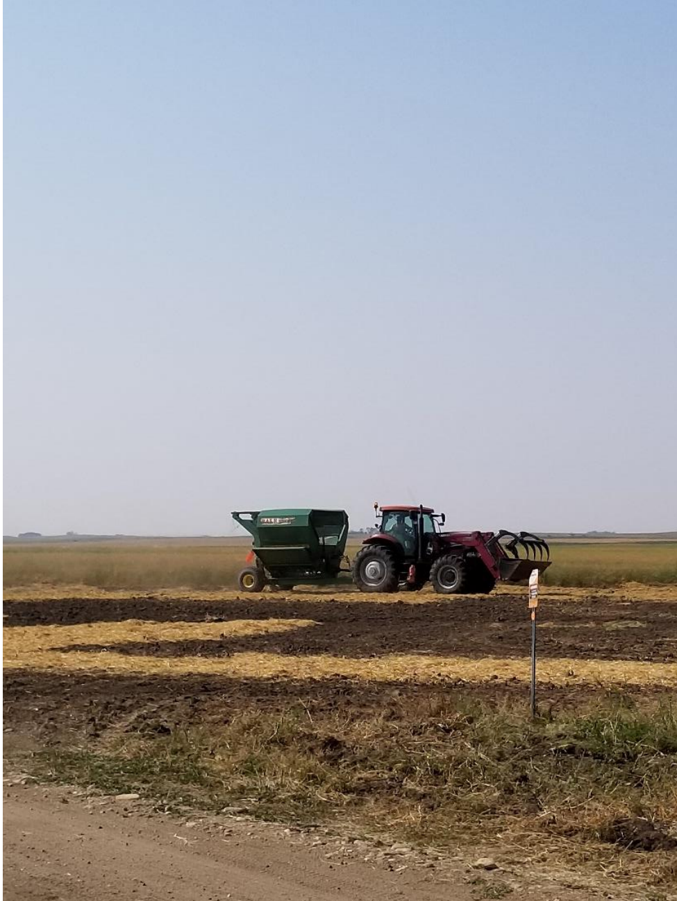
Straw crimping. Straw bale is put through the shredder and sent flying out into ROW.
