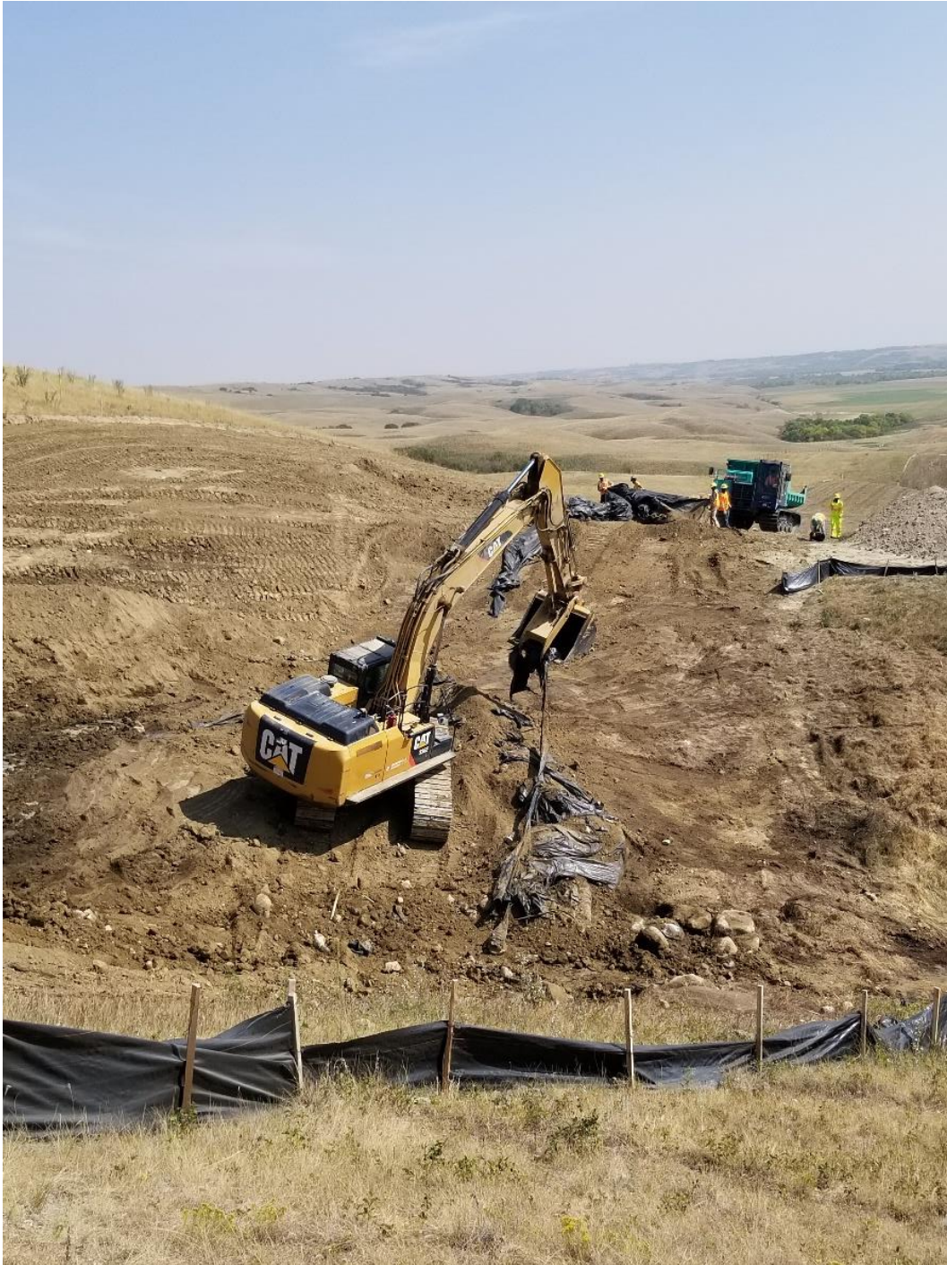
Geo-tech fabric being removed and dug up to be disposed in preparation for re-constructing the slope.
