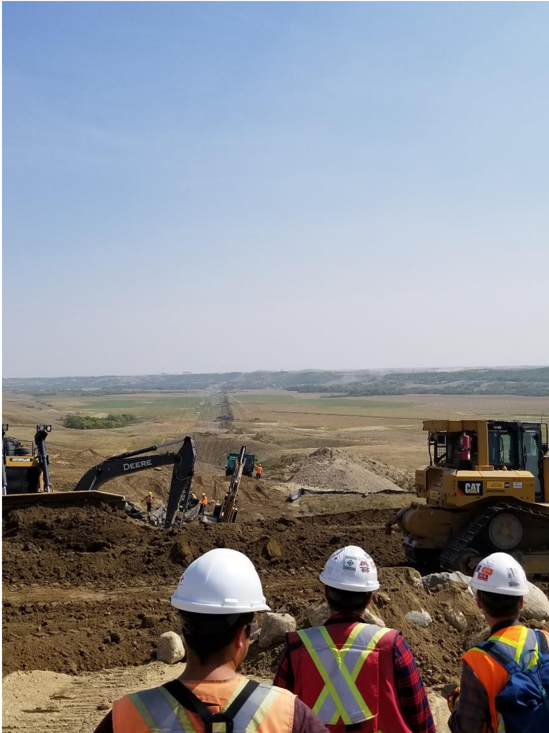
Pasqua Monitors watching equipment put back slope.
