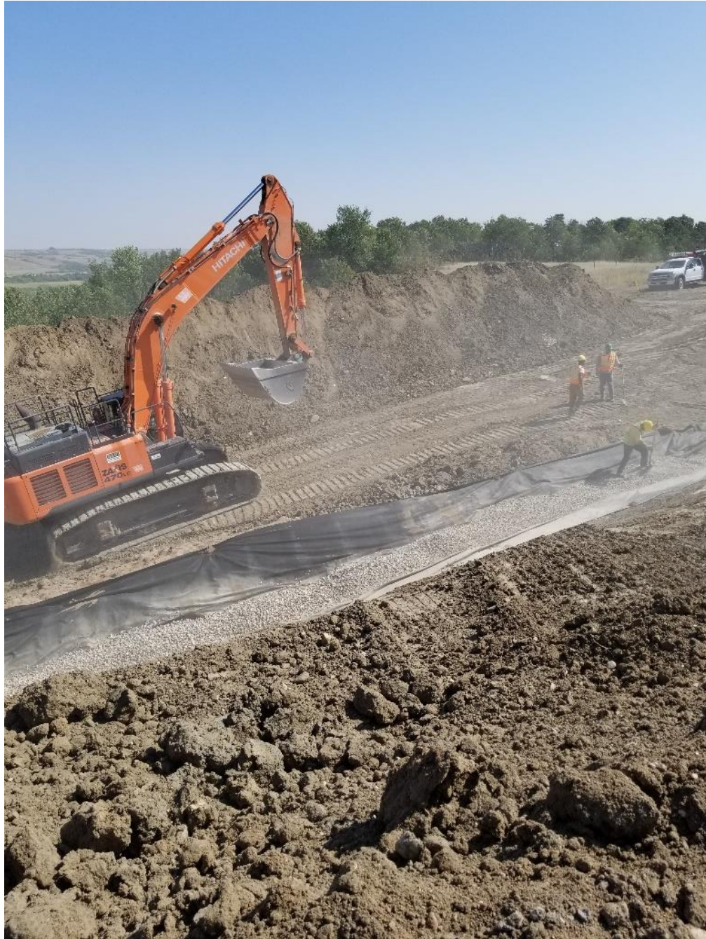
Installation of water drainage at Qu'AppelleValley.
